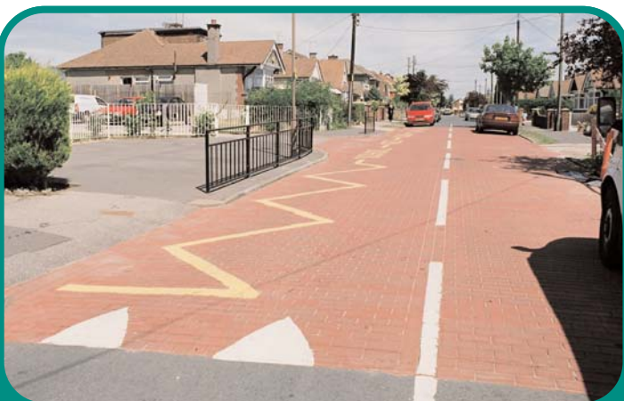
2.1.1. Flat topped road hump with a long plateau for buses
