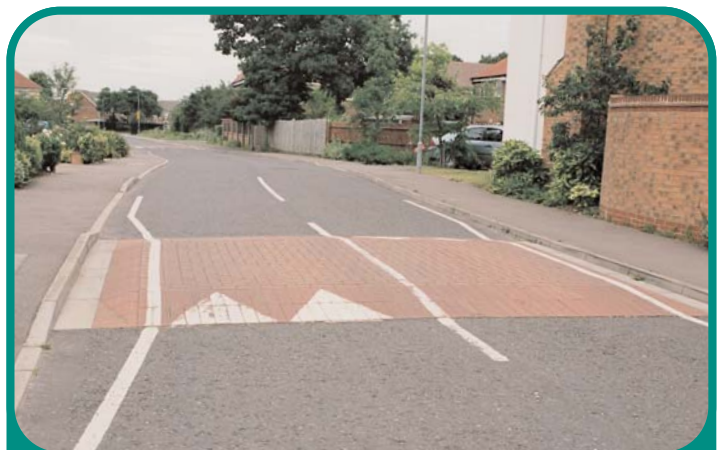
3.1 Flat topped road hump with a short plateau as it is not on a bus route
