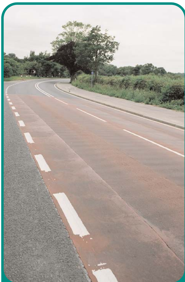
2.2. Rippled rumble surfacing
